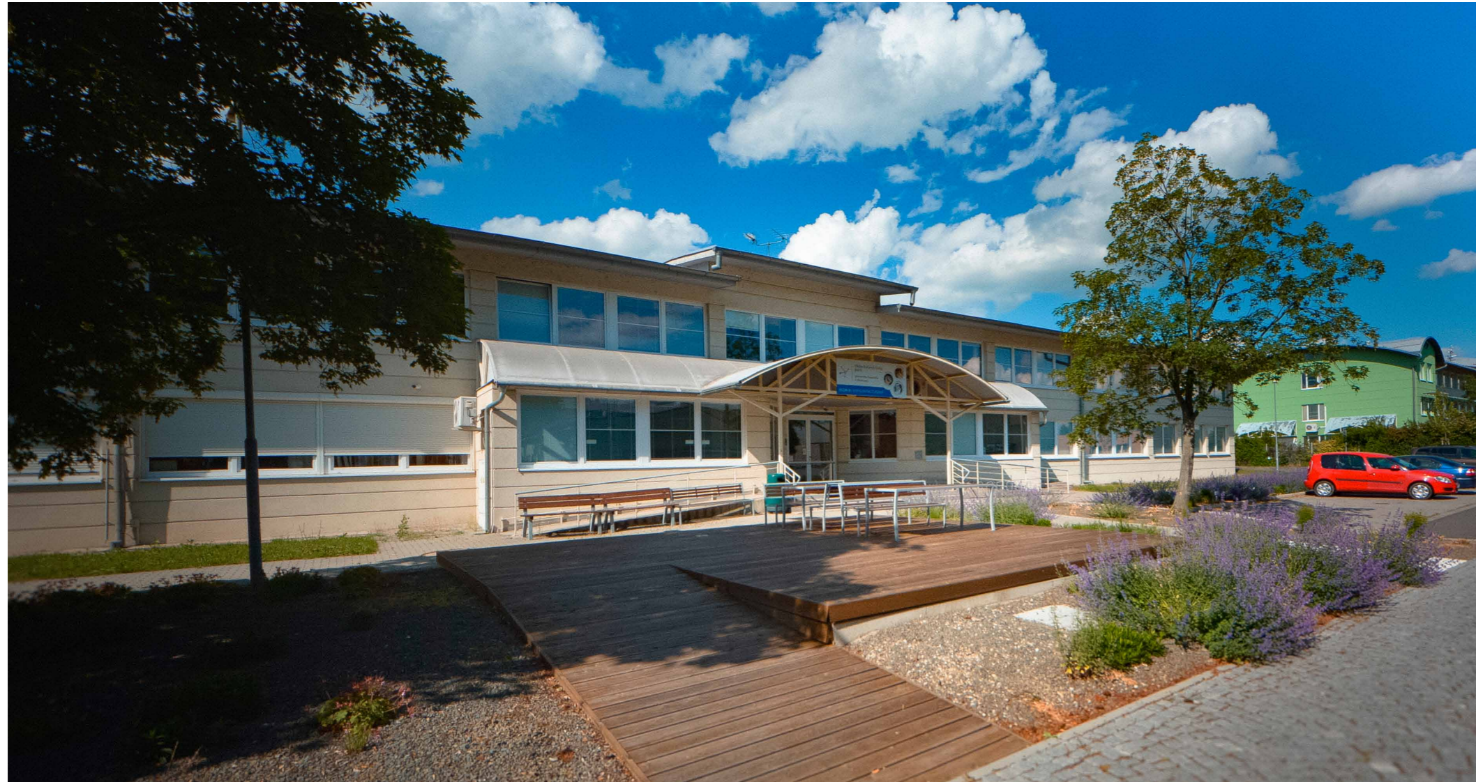
← UP STP building in Block B
