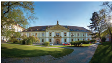
After a costly renovation, UP opens the former Theresian Armoury as its new Central Library and Information Centre.
