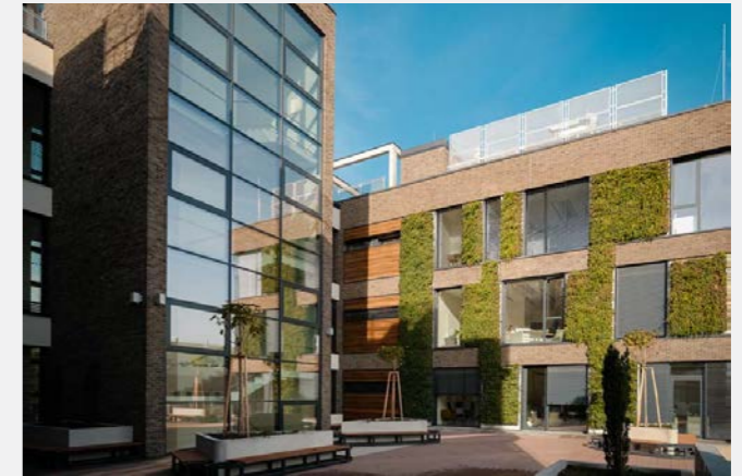
↑ The Envelopa Hub building's façade is adorned with nearly 18,000 plants.
